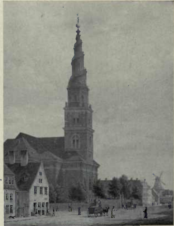
FIRST LATTER-DAY SAINT MEETING HOUSE, COPENHAGEN, DENMARK.
